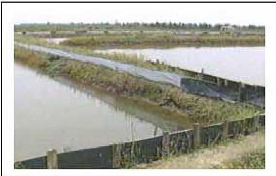
Figure 1: Individual pond crab fence containment. Recommend use of UV stabilise HDPE sheet ~ 400-500mm high, buried into ~ 300-400mm trench, and staked.
